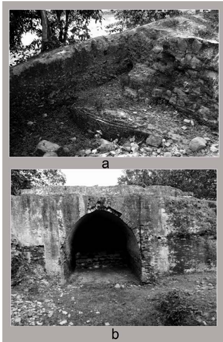
Fig. 18: Excavation in Gaur by ASI: a) A part of a semi-circular bastion like structure; b) Arched guard room with embedded iron chain.
